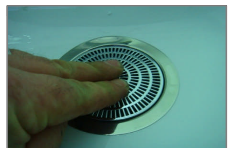
CHECK THAT THE EDGE OF THE MOUNTING FLANGE IS PULLED DOWN AND THERE IS NO SHARP EDGE
