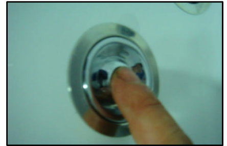
Check action of eyeball by pivoting from side to side. Should be smooth action, not loose.
