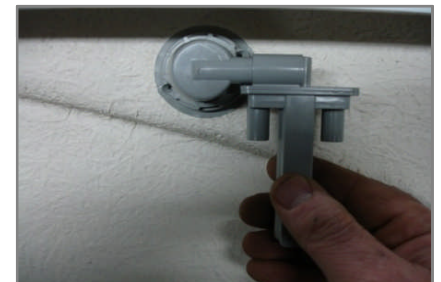
Glue Hartford loop onto spigot, positioning Hartford loop in as close to vertical position as possible
