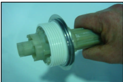
Locate retainer and mounting flange into hole in bath
