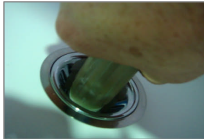
Jet will unlock and ramp out of retainer and become free to remove.
