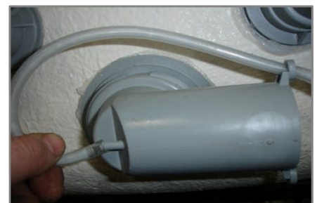
Glue and fit 5mm ID tube as shown feeding through retaining lugs to prevent accidental removal.
