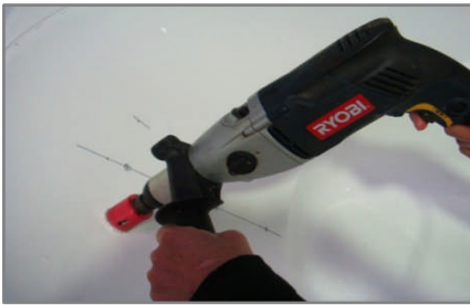
Drill hole through bath wall using 1.5 inch hole saw
