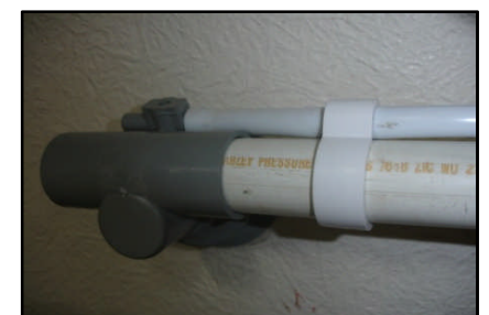
Fit clamping clip to retain pipe
