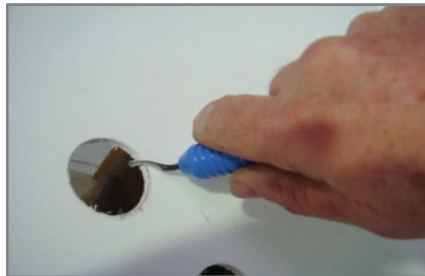
Remove any burr on top edge of hole with deburring tool. A burr could prevent stainless flange sitting flush.
