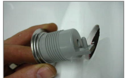
Remove nut from body and pass body through hole.
