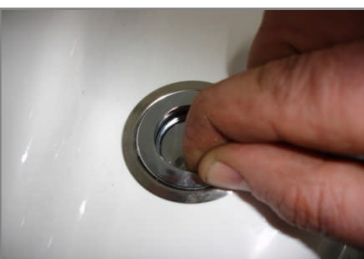
Unclip the air button trim as by twisting in anticlockwise direction as shown
