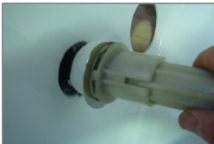
Locate flange and stainless steel mounting flange into hole in bath
