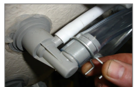
Fit clamping clip to retain pipe
