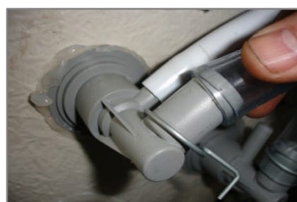
Push 19mm flex pipe on barb spigot.
