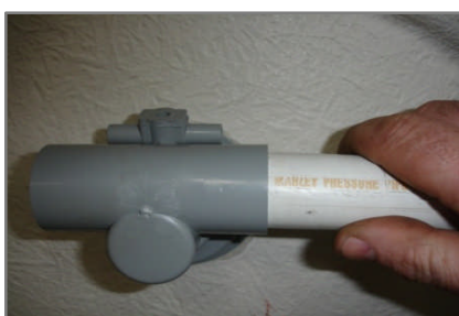
Glue 25 pressure pipe into sockets
