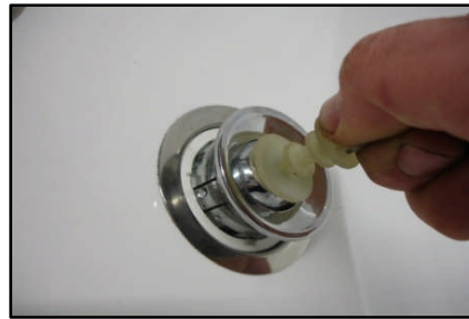
Pull out with a firm action. Remove tool from centre of jet face
