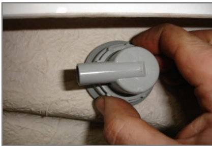
Refit nut and hand tighten, pulling the conical flange on the nut down onto the bath wall.
