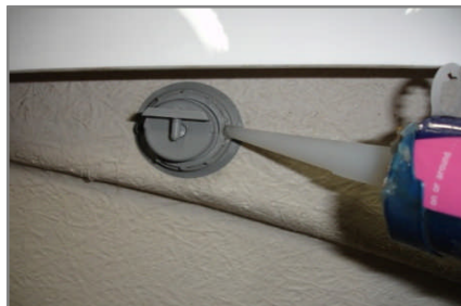
Inject silicone through one of the injection holes in the nut until it oozes out the opposite hole.
