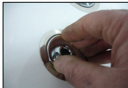
Insure Jet clips fully home and locked in place, CHECK EYEBALL IS NOT LOOSE
