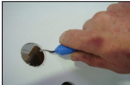
THERE MUST BE NO BURR ON EDGE OF HOLE, a burr could stop the mounting flange sitting down flush
