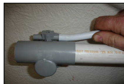
Push 19mm flex pipe on barb spigot.
