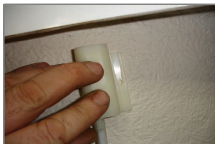
Stick Hartford loop less than 30mm from the top of the bath rim. SEE MAX DISTANCE ON SPEC SHEET.
