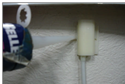
Apply silicone bead to each side of Hartford loop to ensure component sticks to bath permanently.
