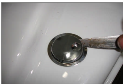
Remove cap by lifting under edge as shown.
