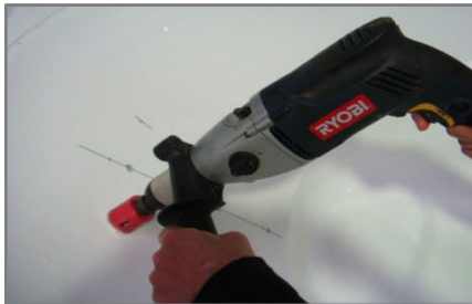
Drill hole through bath wall using 2 inch hole saw
