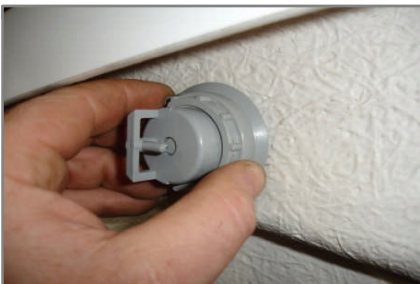
Refit nut and hand tighten, pulling the conical flange on the nut down onto the bath wall
