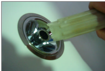
Using Installation Tool 500109 insert drive legs in slots at bottom of jet and rotate anticlockwise
