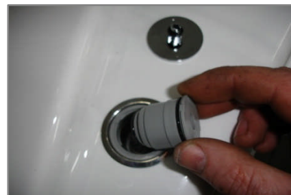
Pick out centre piece as shown. Internal components can now be accessed for servicing.
