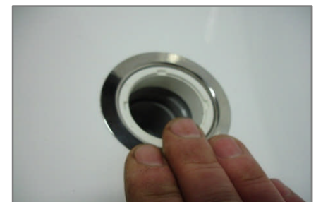
CHECK THAT THE EDGE OF THE MOUNTING FLANGE IS PULLED DOWN AND THERE ARE NO SHARP EDGES
