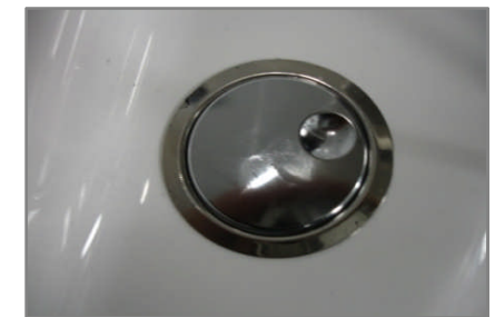
Inspect and replace if required, re-assemble unit
