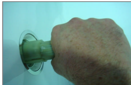
Using Tool MT0168 tighten retainer into elbow. Max torque 14nm
