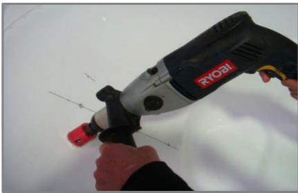
Drill hole through bath wall using 3 inch hole saw
